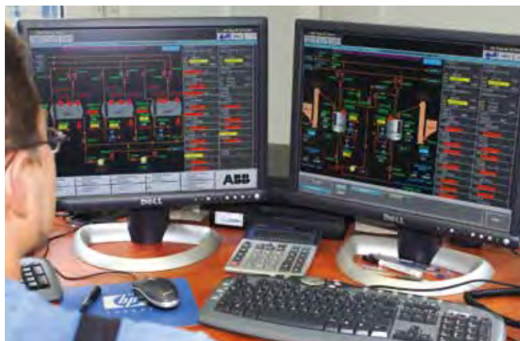
Figure 1.4. DCS system for the Plock site ORBITON modified bitumen production (photo by ORLEN Asphalt)
